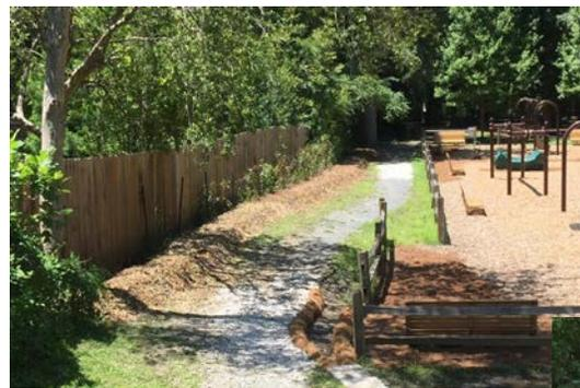
Equally important, they constructed a wood chip berm along the fence line. This will dramatically improve the flow of water through the park and have a meaningful impact in preventing erosion and minimizing further damage to vulnerable landscaping.
